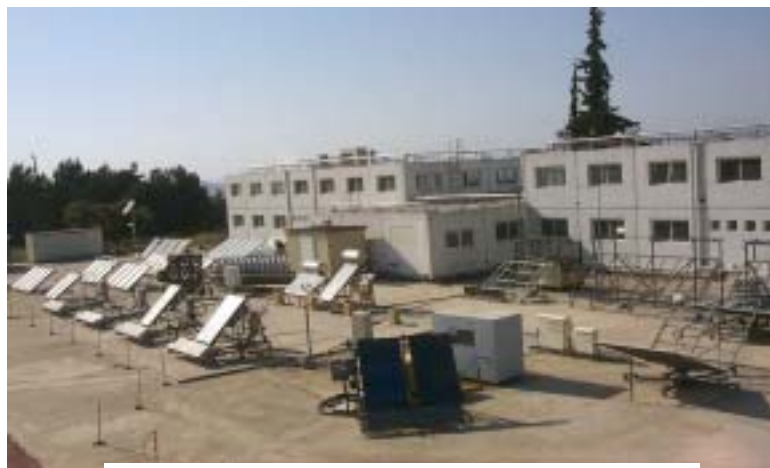
General view of the outdoor measurement and testing facilities
